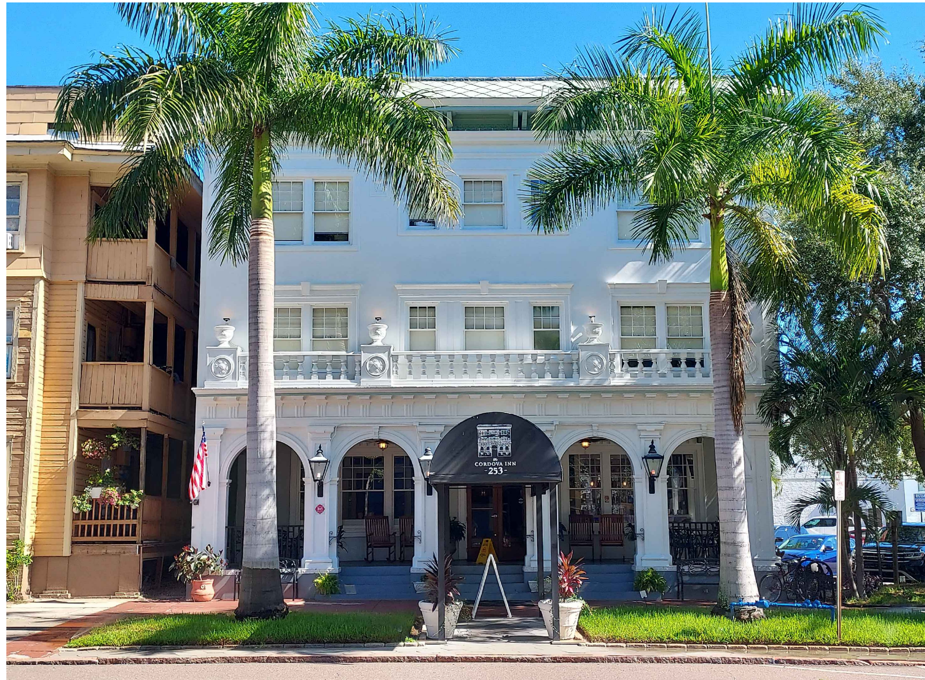
P1 Photo #1 - Existing South Elevation NOT TO SCALE
