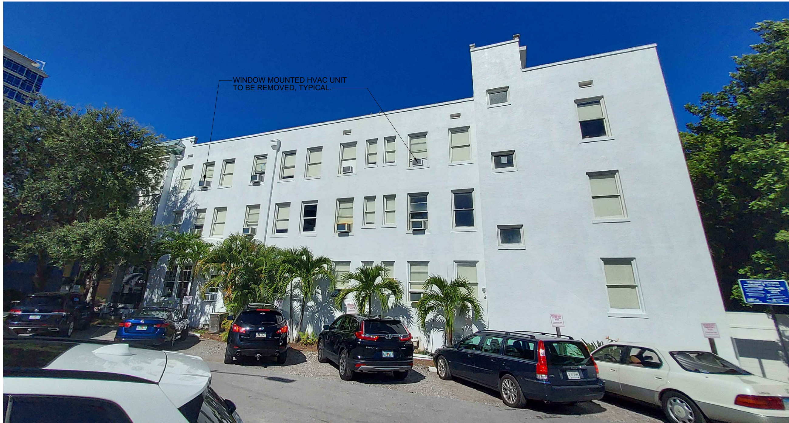
P2 Photo #2 - Existing East Elevation NOT TO SCALE
